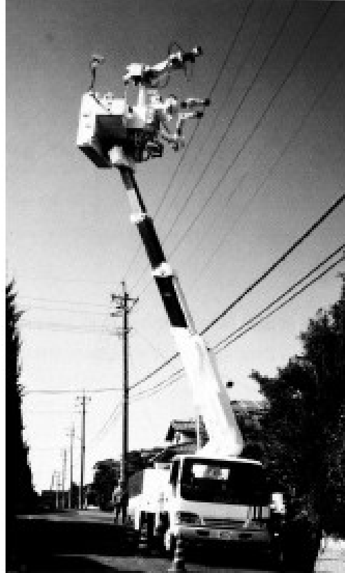
Figure 15.9: The "Hot-Line Telerobot System" from Kyushu ELeetric Power Co. A teleoperated robot repairs a high-voltage power line (left). The operator's interface to the system (right). (Courtesy of Blake Hannaford with permission of MIT Press. Reprinted from K. Goldberg, The Robot in the Garden , Cambridge, MA: The MIT Press, 2000.)
